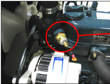
Coolant Temperature Sensor (above alternator)
