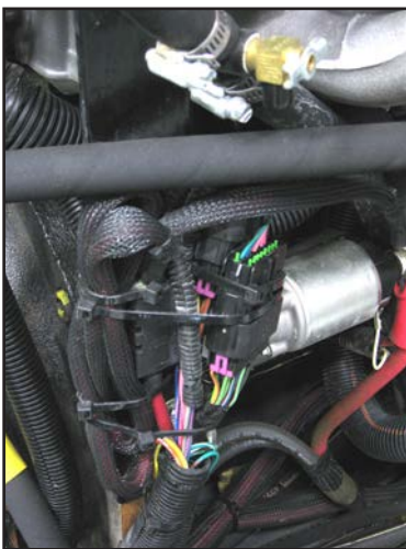
X1 and X2 Electrical Connectors
