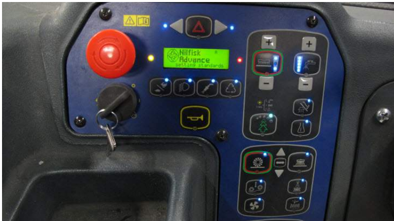
Control panel appearance with CAN Bus failure
