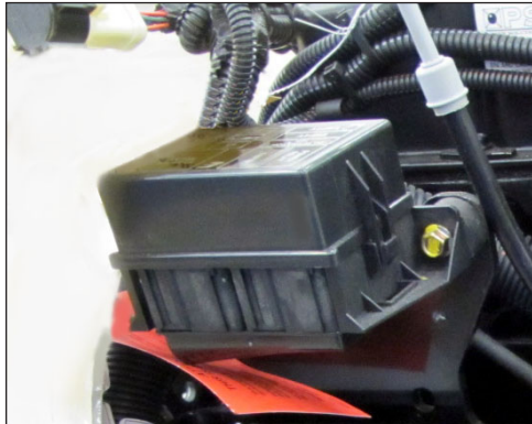
Engine Fuse Box
