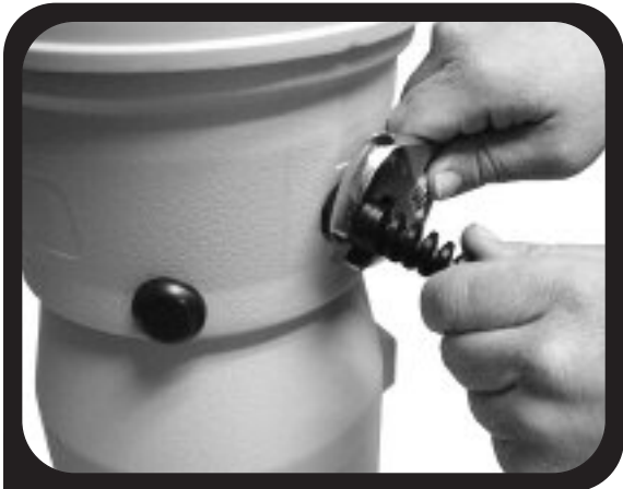
7a. With crescent wrench holding nut unscrew the strain relief.
