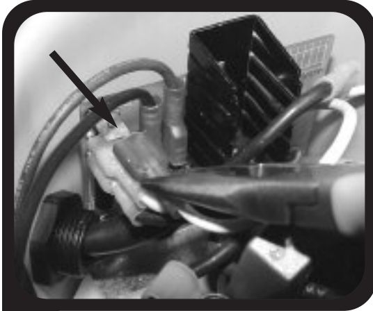
4. Locate white wire from receptacle and remove from BCM.
