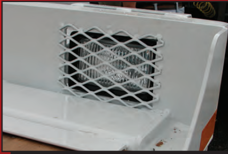
Loading lights in safety bulkhead
