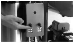
Safety on/off switch for the burner and the pump are easily accessible.
